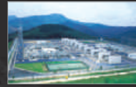
Electro Electric Systems Division
